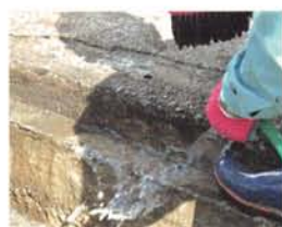
1 既存側溝の清掃
